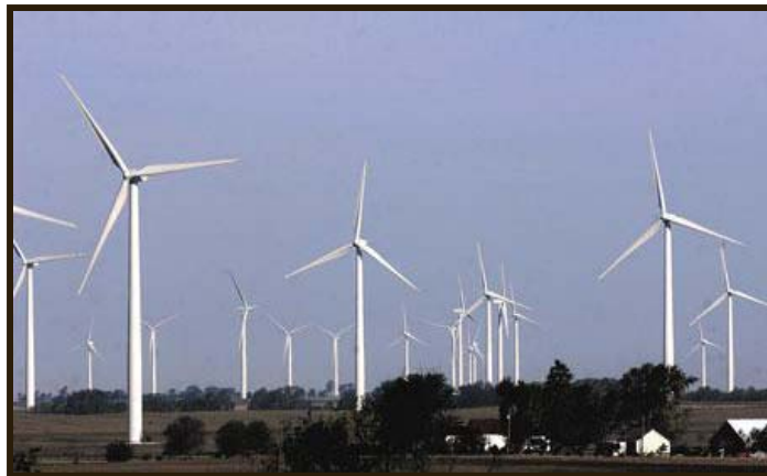
Wind turbine propellers that are used to generate electricity.
